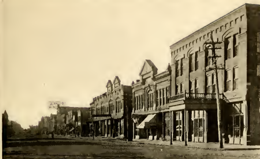
Meridian Street looking South, Portland, Indiana.
